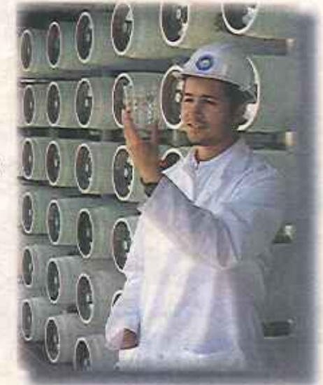
Photo courtesy of West Basin Municipal Water District
